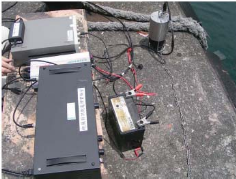
Figure 1.20: Equipment setup at transmitter site [45]
